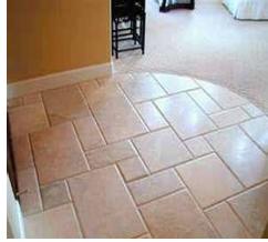
Laid in Offset Pattern
